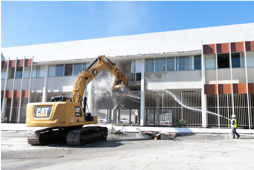
Demolition begins for the shuttered San Pedro Courthouse | Genton Cockrum Partners
